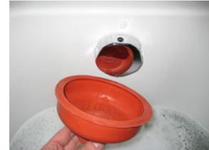
To drain the tub, I just remove the plunger and open the plug by turning the handle.
